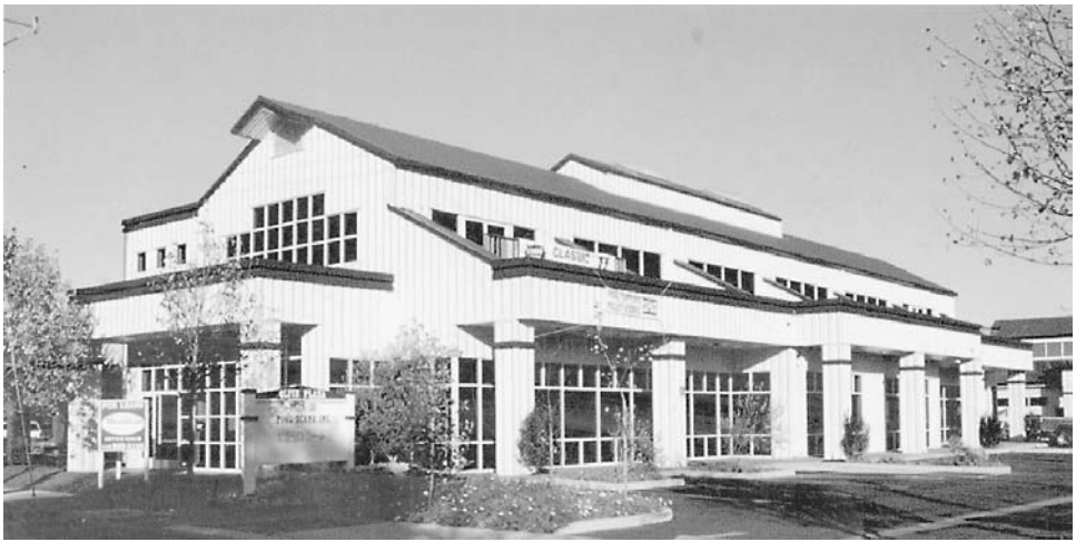
FIGURE 1.4 Metal building system in a commercial application. (Photo: Bob Cary Construction.)
